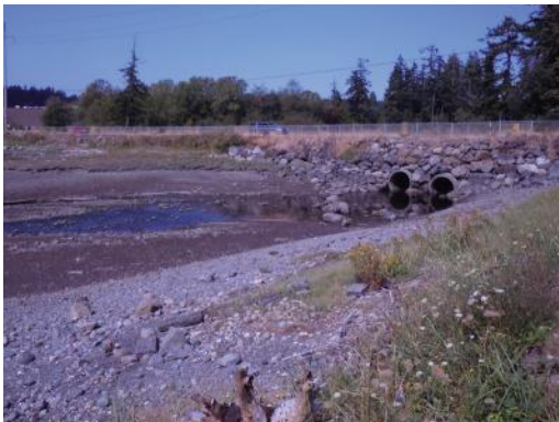
Figure 5.1 Existing Bucklin Hill Road culverts at Clear Creek estuary slated for replacement in 2012. (Image by BCRA)
