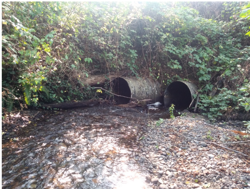
Figure 2 Culvert inlet
