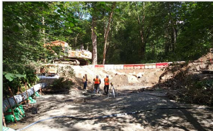
Culvert removed
