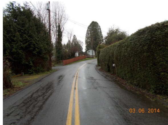
Picture 4 -Nokomis Road SE 700' south of SE Olympic Drive (Looking south)
