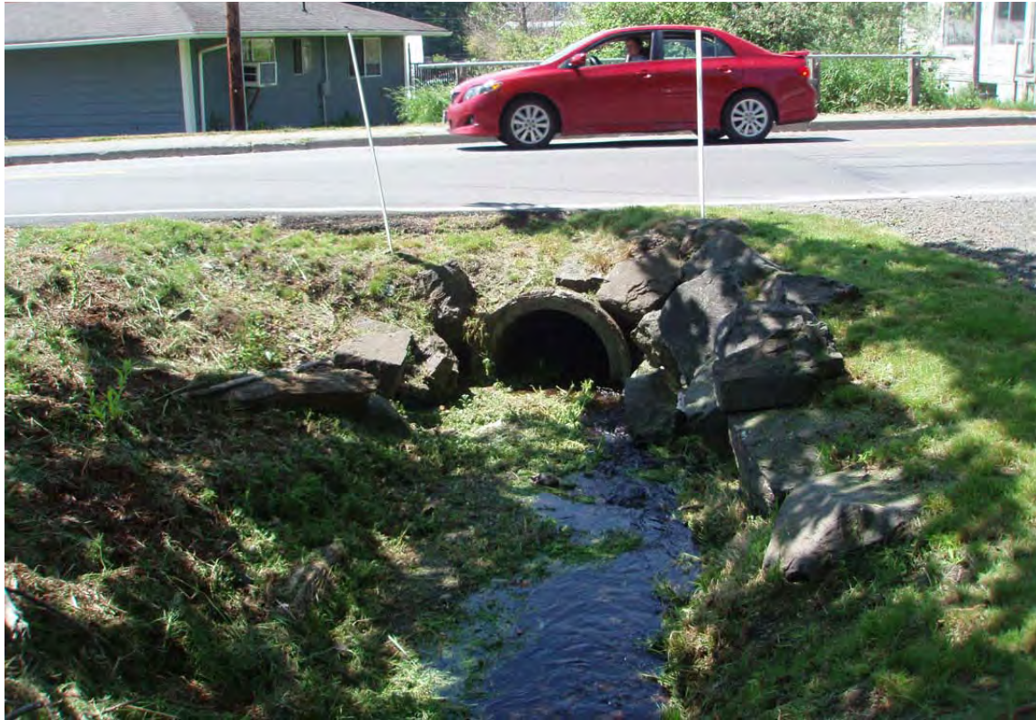
Photo 16. Riparian zone surrounding undersized culvert at 8th Avenue NE, facing downstream
