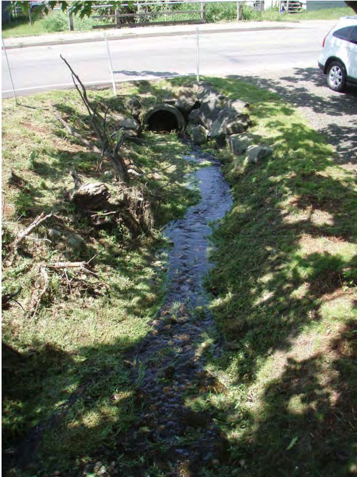
Photo 1. Undersized culvert at 8th Avenue NE, facing downstream
