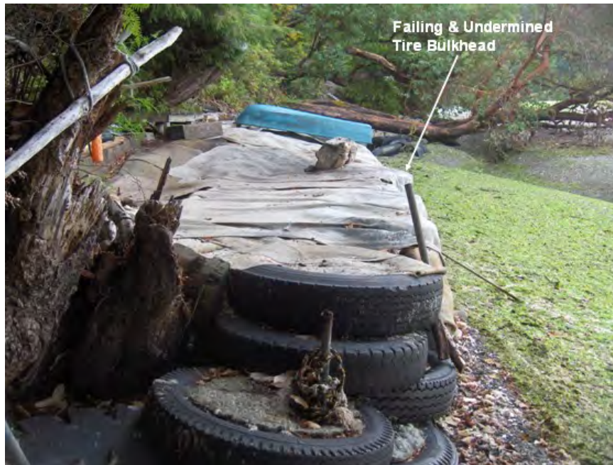
Figure 7. Scrap tire bulkhead constructed to protect upland from erosion
