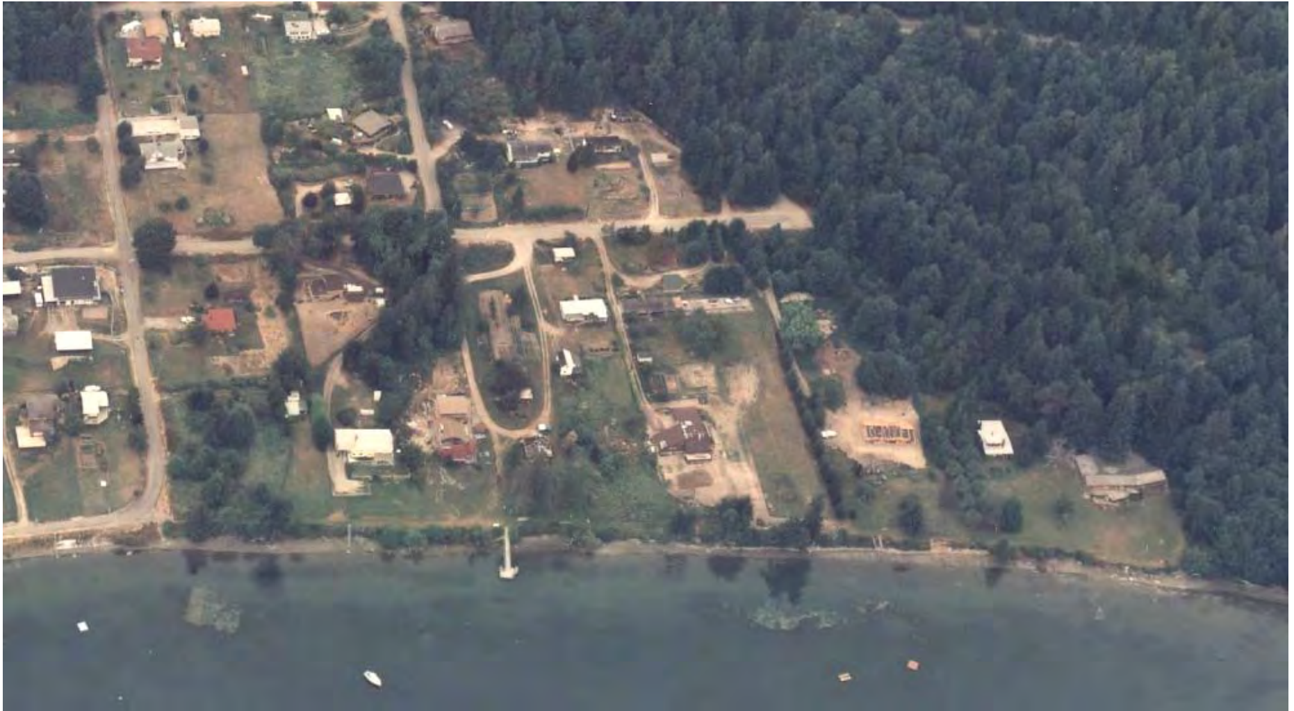
Figure 2. Von Geldern Cove site. Image enlarged from 6/27/77 shoreline oblique by WA Dept. of Ecology. Williams house (red roof, near center) was recently constructed with cut visible in landward portion of yard and apparent fill near marine bank.
