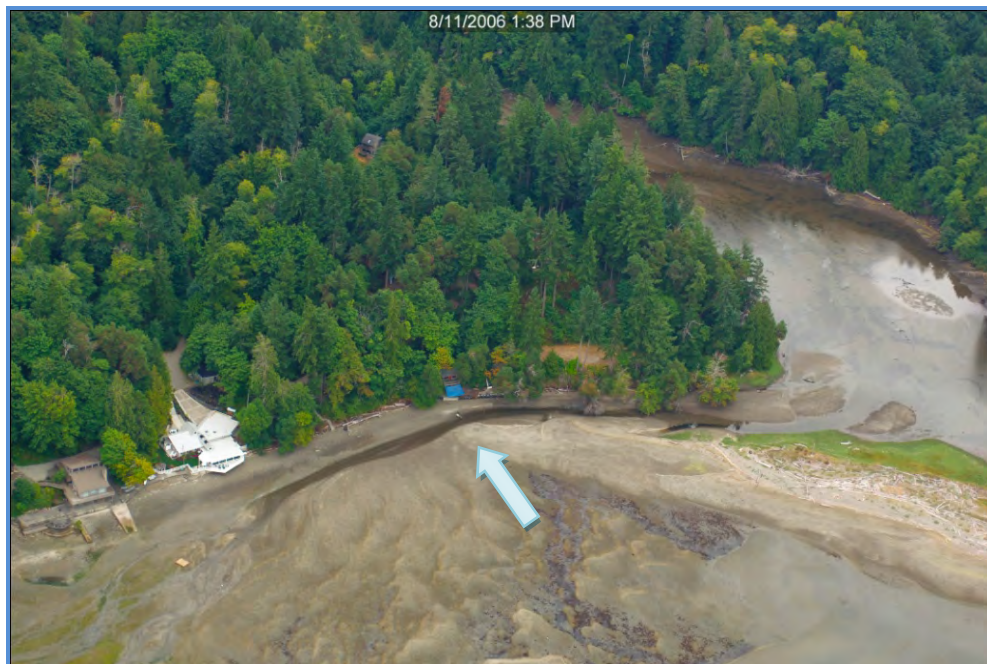
Figure 7.4. Aerial photo (DOE 2006) showing the bulkhead, lagoon, and tidal channel before channel reroute in 2009.
