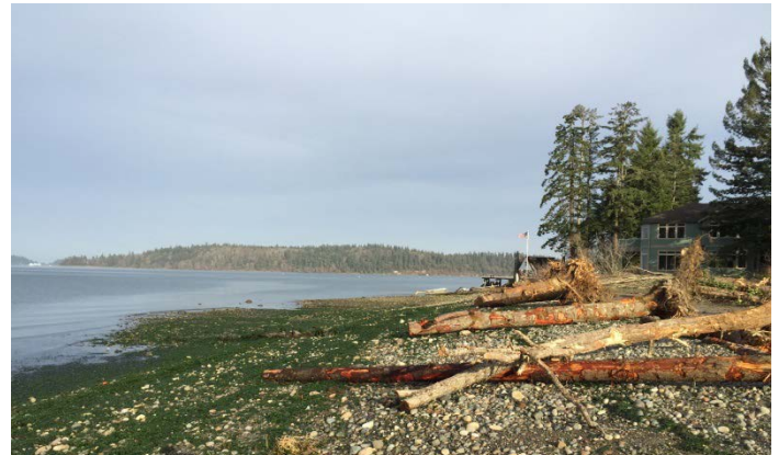
Area where bulkhead was removed at the northern end up the project area
