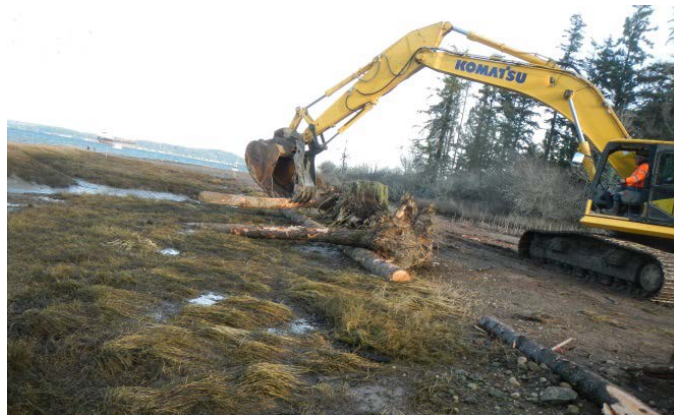
Excavator placing large wood with root wads after fill was removed
