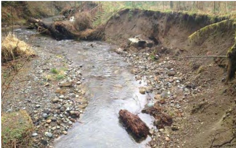
Figure 61. Photo of incised channel segment on Dickerson Creek downstream of failed log weirs (view downstream). Note box at toe of right bank is exposed septic basin. Photo by Tim Abbe, NSD (2/12/2013).
