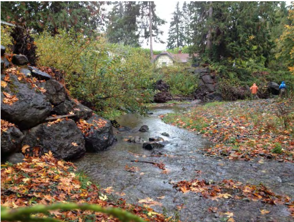
Figure 54. Photo of incised channel and riprap bank protection along the left bank downstream of Northlake Way. Photo taken in Oct. 2012 by Shawn Higgins (NSD).
