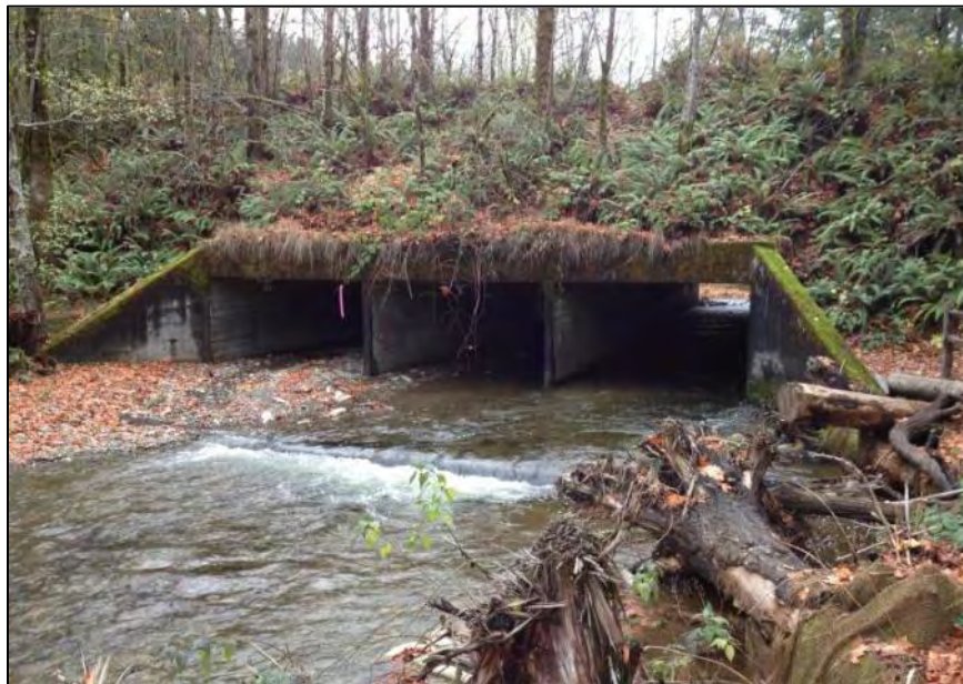
Figure 50. Photo of the triple box culvert at NW Golf Club Hill Road (view upstream). Photo taken November 2012 by Shawn Higgins, NSD.
