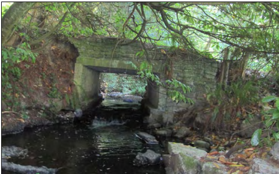
Figure 58. Photo of partial barrier to fish passage in Kitsap Creek at RS 2400 (view upstream). Photo taken August 2012 by Steve Todd, Suquamish Tribe.
